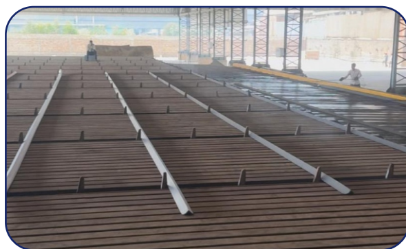
AUTOMATIC COOLING BED
